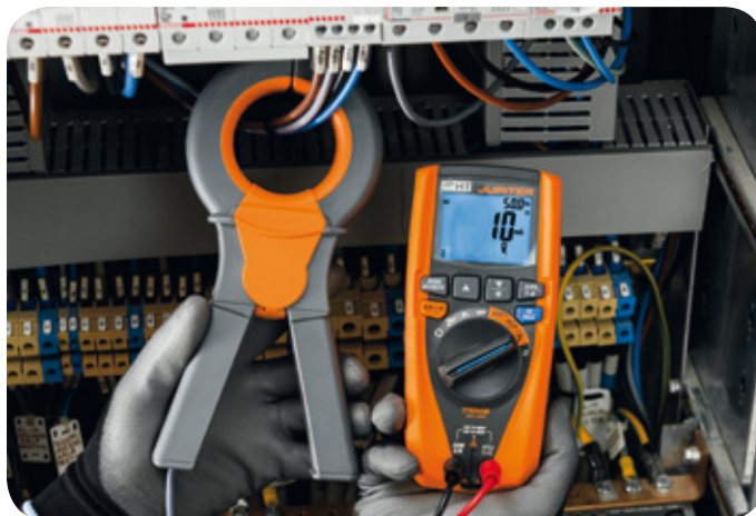
Leakage current measurement.
