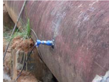
Installation Drawing of Insertion Flow Transducer
